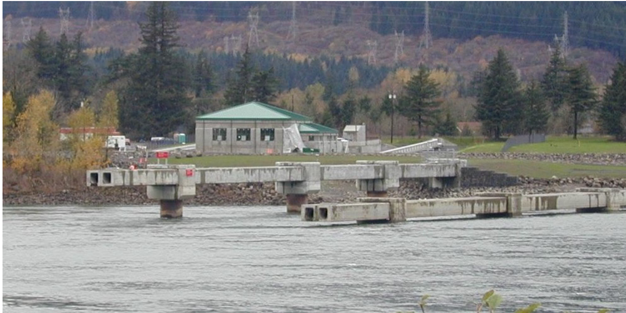
Figure 6-13. JBS Outfall Piers
