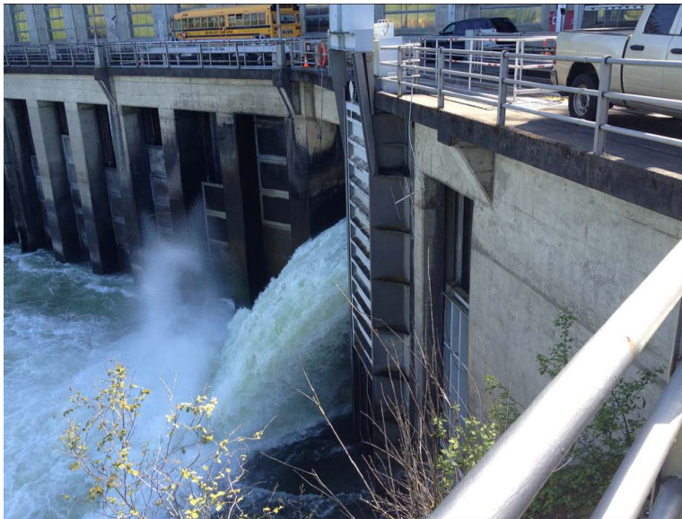
Figure 6-7. B1 ITS Outfall Pass-Through Antenna
